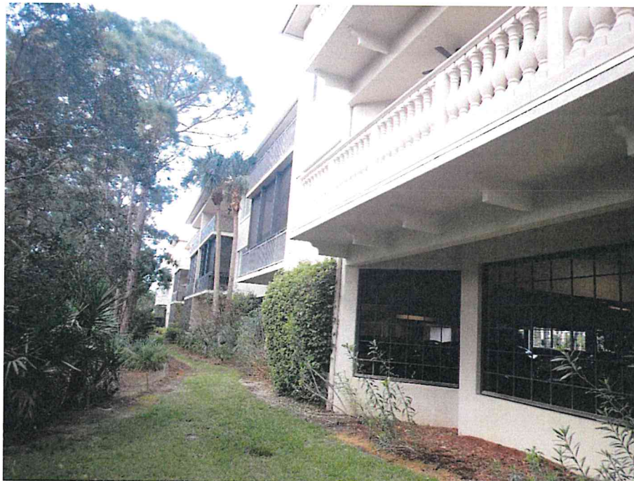
4. View of the rear of the building looking southwest.
