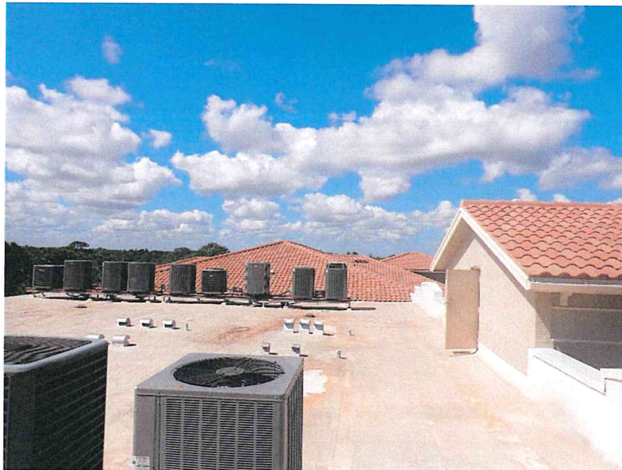
10. View of the roof systems looking southwest.
