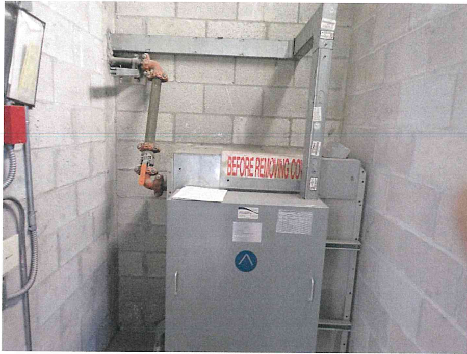
9. View of the elevator room.
