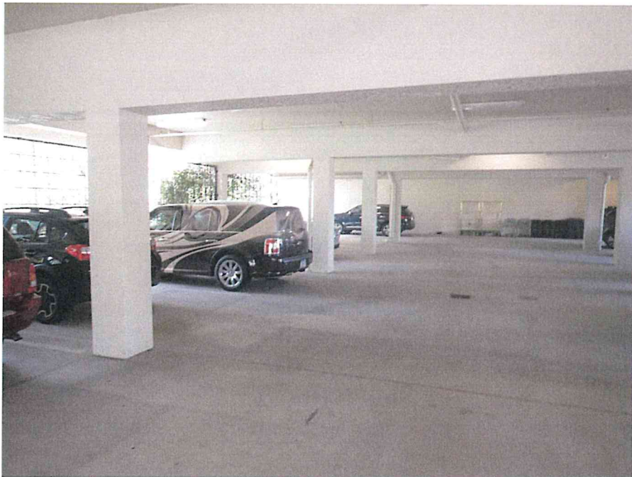
6. View of the interior of the parking garage.
