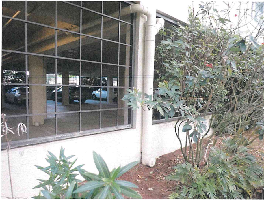
5. View of the parking garage.
