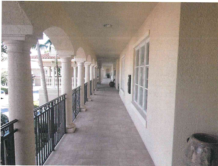
14. View of the typical tile-covered walkway.
