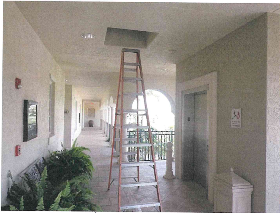
15. View of the 3 rd floor elevator and roof access opening.
